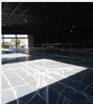
FIGURE 4: The influence of curing illustrated when using a curing cover where the wrinkles have not been removed. The wrinkle locations will show when the slab is polished.
