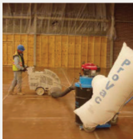
FIGURE 8 - Form contraction joints with an early-entry power saw using a dry-cut blade with a vacuum to remove saw cut residue, otherwise a stain from the residue will show when the concrete is polished.
