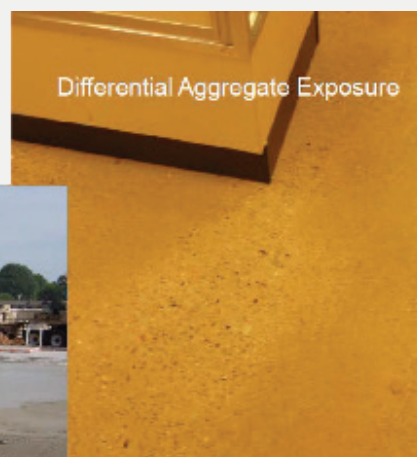
FIGURE 1 - Bump Cutting: Differential aggregate exposure due to bump cutting, scraping the paste off the high spots and depositing it in the low spots. When polishing, the aggregate in the high spots will be exposed first.
