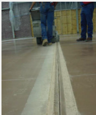
FIGURE 3 - Residue and Scratches Below Plate: The effect of saw cutting is shown on the polished surface when the saw cut residue is not removed by vacuum.
