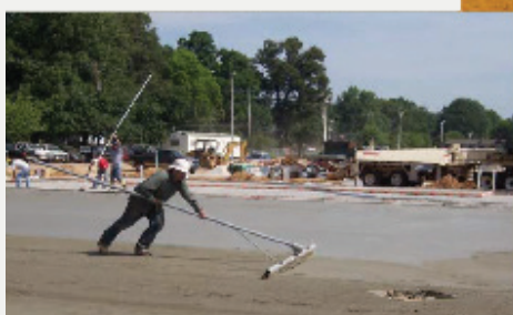
FIGURE 2 - Minimize Hand Finishing: Difference in surface finish density results from hand versus machine finishing. Note the difference in the polished surface
