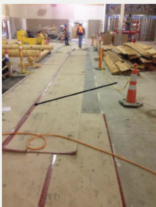
FIGURE 5 - Discoloration from Tape Lines: The impact of protection is clearly shown by the discoloration of the tape lines after the floor is polished. What everyone thought would provide excellent protection, still turned out to show through on polishing. Be very careful with even the smallest of details when providing protection.
