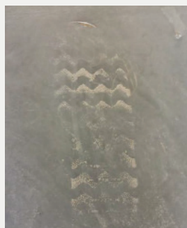
FIGURE 6 - Footprints Seed Aggregate: Footprints push aggregate lower, bringing more paste to the surface and this difference can be seen during polishing.
