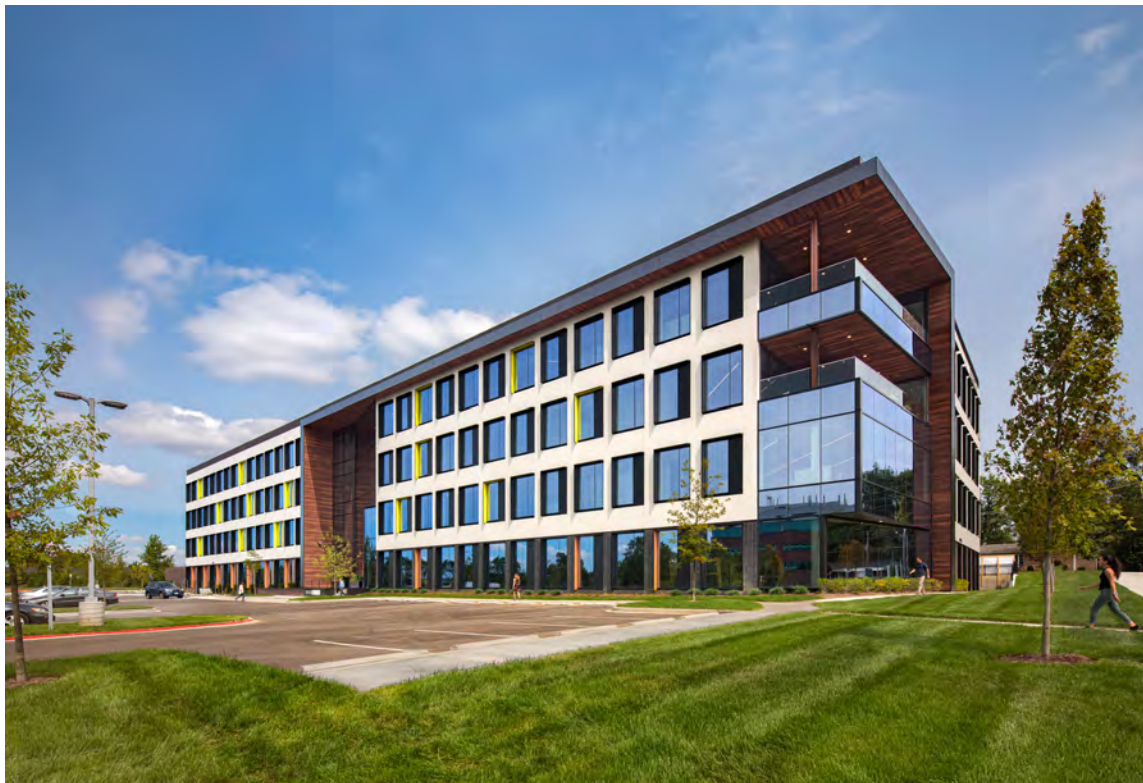
Edge @ BRDG, Concrete Strategies, St. Louis, MO
