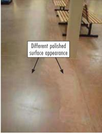
The photos illustrate the differences in a polished surface along a slab construction joint. Near the joint, the slab was finished with a handheld trowel. Away from the joint, the surface was finished with a walkbehind trowel. A distinct change in surface density was produced within an arm's length of the joint.
