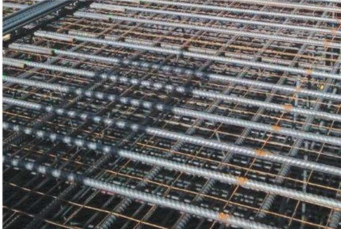
Welded wire reinforcement placed over top bars in a mat foundation so workers can safely perform their tasks. (Photos courtesy of Tim Manherz-- TAS Commercial Concrete Construction, Houston, TX)
