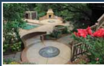
CAST-IN-PLACE, SPECIAL FINISHES Under 5000 SF – 1st Place Project: Pott Hardscape Contractor: Tom Ralston Concrete
