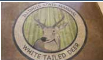
POLISHED Over 5000 SF – 1st Place Project: Kennekuk County Park Environmental Education Center Contractor: Creative Construction By Design
